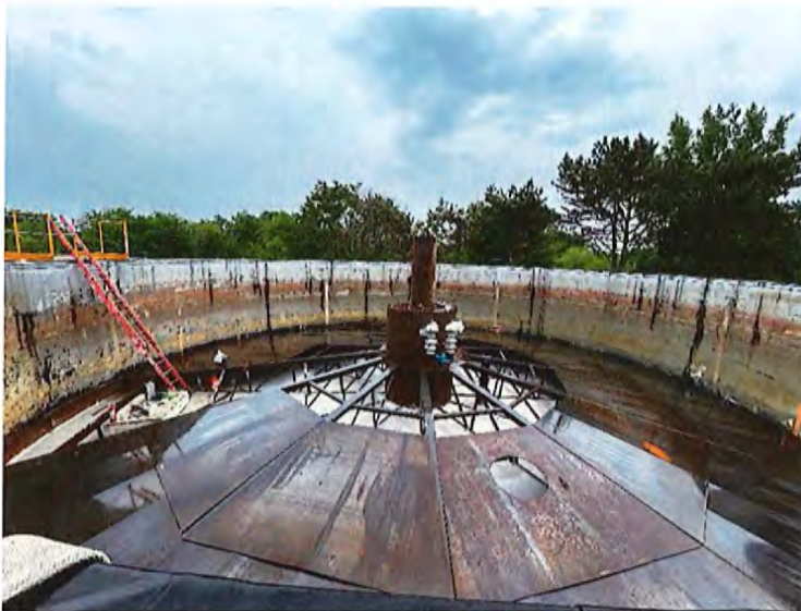
Figure 1: Welding on Digester Cover
